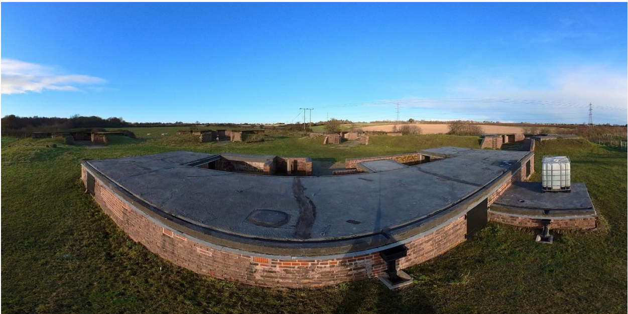
Plate 22-5-3 Heavy Anti-aircraft gunsite (1019186) with the command post in the foreground, viewed from southeast (taken with a 360° camera).
